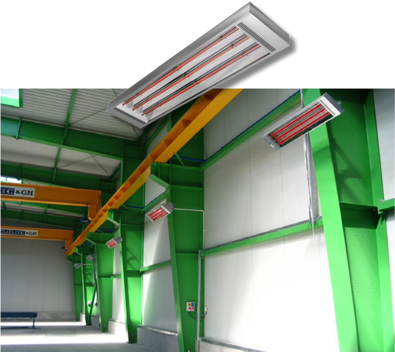
Energolnra Industry provides an energy efficient heating for most applications and working environments with high ceiling heights, approximately 3-40 m. Heat accumulation in floors, walls and other surfaces means that the air temperature can be lowered, giving 25-50% energy savings and yet achieving the same warmth comfort.
