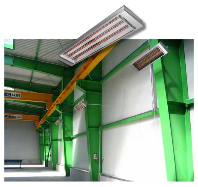
**EnergoInfra Industry** provides an energy efficient heating for most applications and working environments with high ceiling heights, approximately 3-40 m. Heat accumulation in floors, walls and other surfaces means that the air temperature can be lowered, giving 25-50% energy savings and yet achieving the same warmth comfort.
